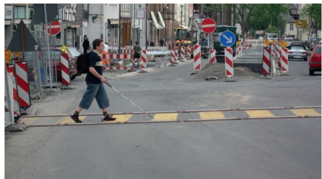
1 | Tactile strips at a provisional crossing in Marburg
